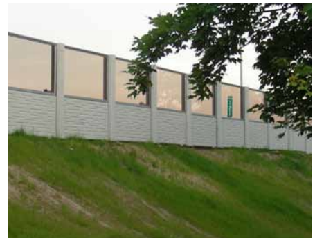
COLUMBUS, OH - ACRYLITE® SOUNDSTOP NOISE BARRIER PANELS
