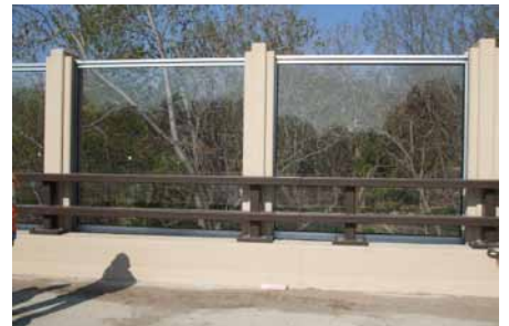
CROSTOWN, MN - ACRYLITE® SOUNDSTOP NOISE BARRIER PANELS
