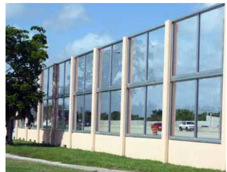
MIAMI, FL - (ALUMINUM) READY-FIT FRAMES INSTALLATION
