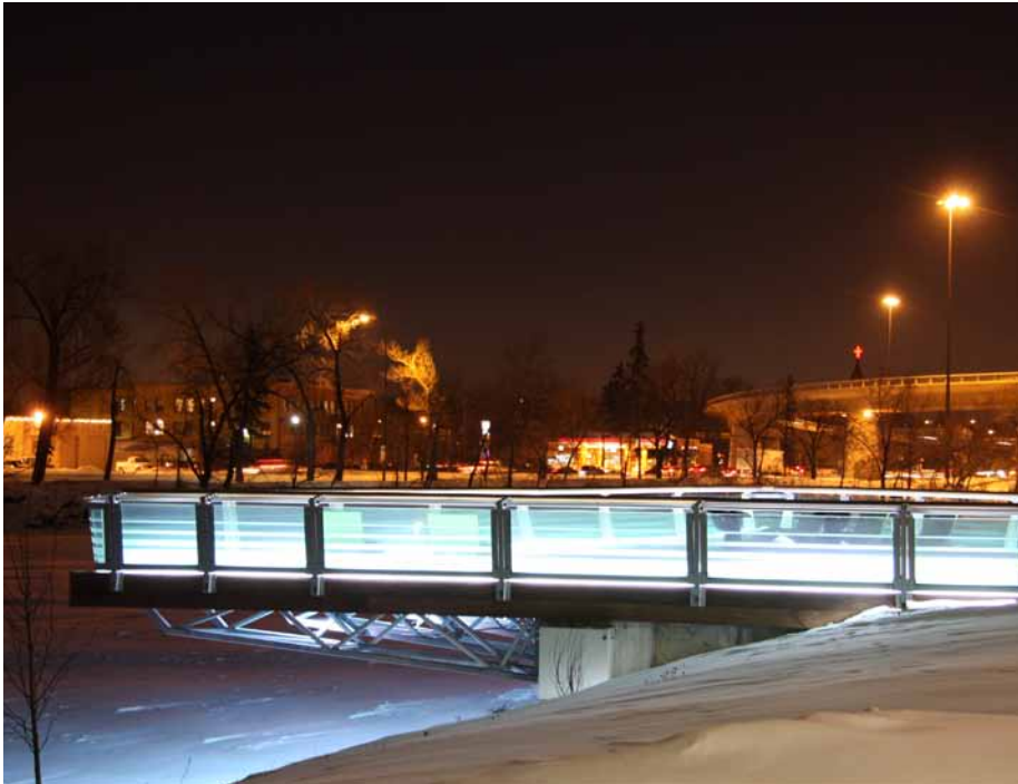
CALGARY, AB - ACRYLITE® SOUNDSTOP NOISE BARRIER PANELS
