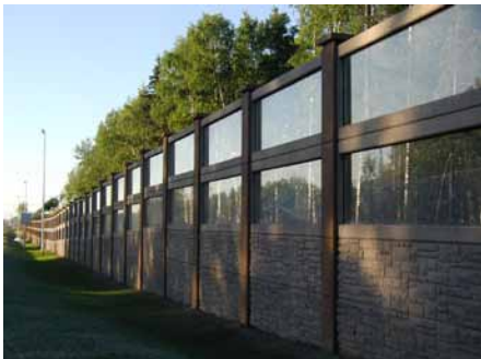
ANCHORAGE, AK - ACRYLITE® SOUNDSTOP NOISE BARRIER PANELS
