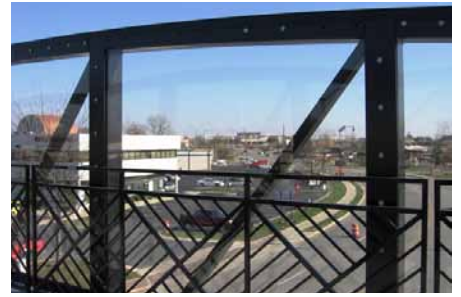
CARMEL, IN - ACRYLITE® SOUNDSTOP NOISE BARRIER PANELS
