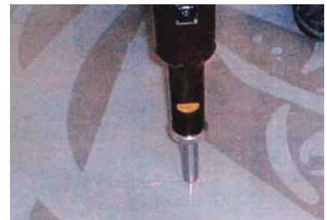
POINT 2 - CENTER IMPACT WITH CONCRETE TESTING HAMMER
