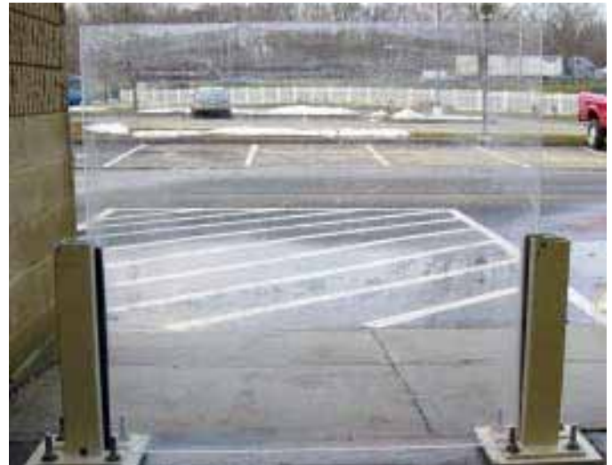
4. AFTER WATER RINSE WITH 2,300PSI PRESSURE WASHER
