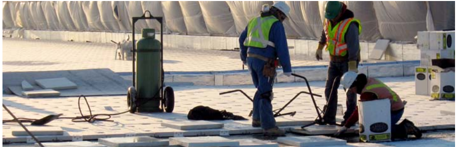
PLACING A SLAB USING LIFTING CLAMP
