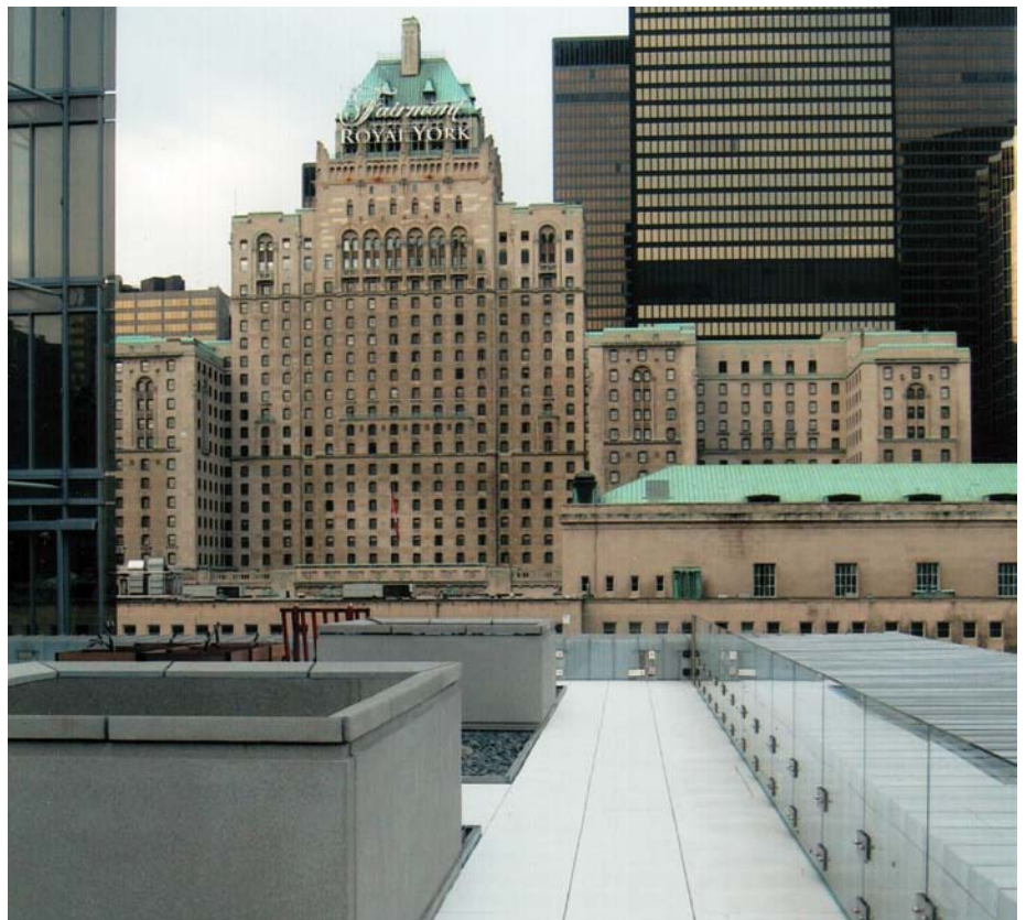
TORONTO, ON - WHITE SOLAR REFLECTIVE ROOF PAVERS
