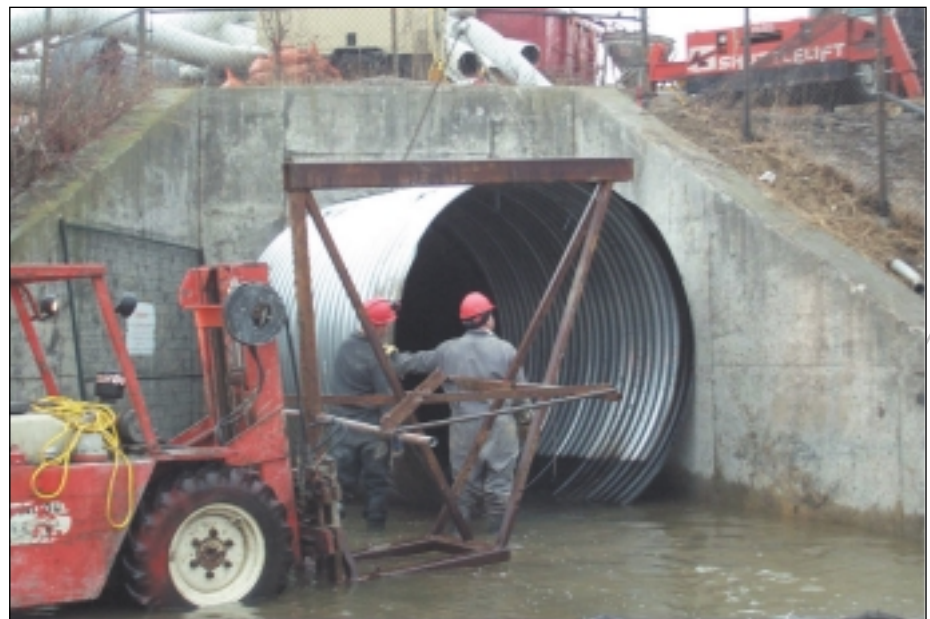
Insertion of the Re-line pipe into the host pipe.
