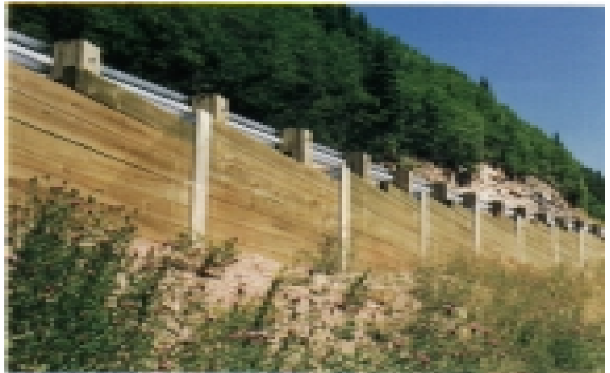
Finished wall installed.
