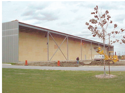
Temporary hoarding in place to keep out the elements during construction.
